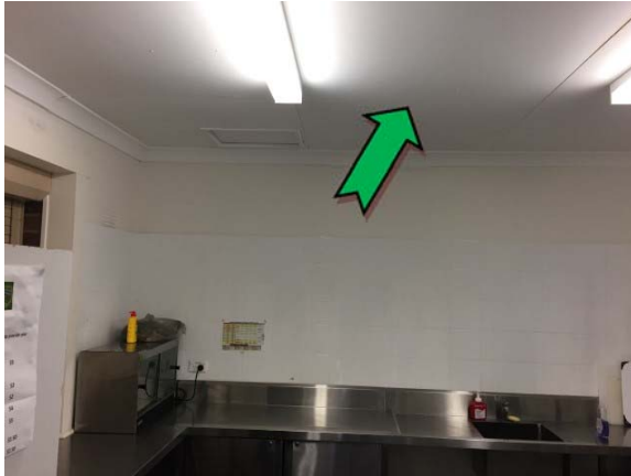
Photo 7. Interior, canteen, ceiling – assumed non asbestos-containing fibre cement sheeting.
