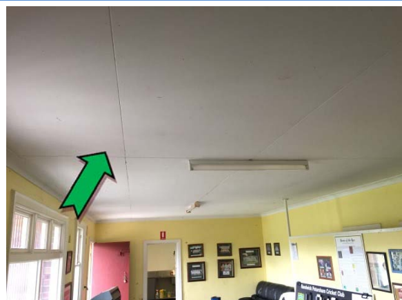
Photo 6. Interior, clubroom, ceiling – non asbestos-containing fibre cement sheeting.
