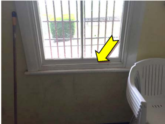
Photo 13. Interior, window frames – lead-containing white upper paint system.
