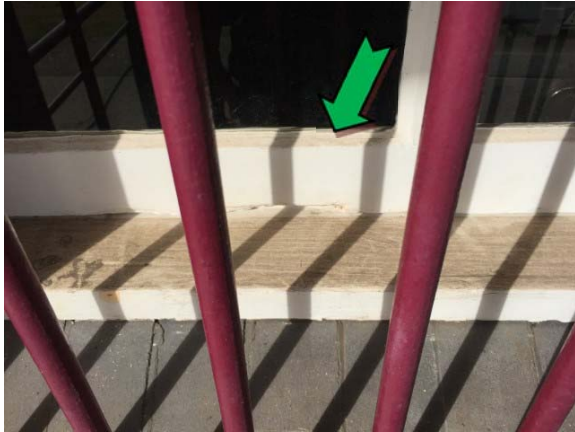
Photo 1. Exterior, ground level, north-east elevation, window frames – non asbestos-containing window caulking.
