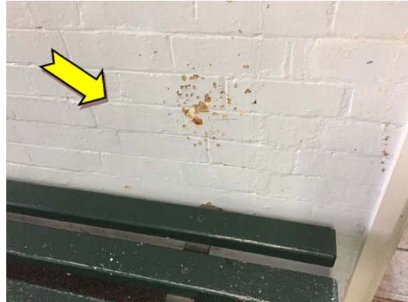
Photo 14. Interior, walls – suspected lead-containing white upper paint system.
